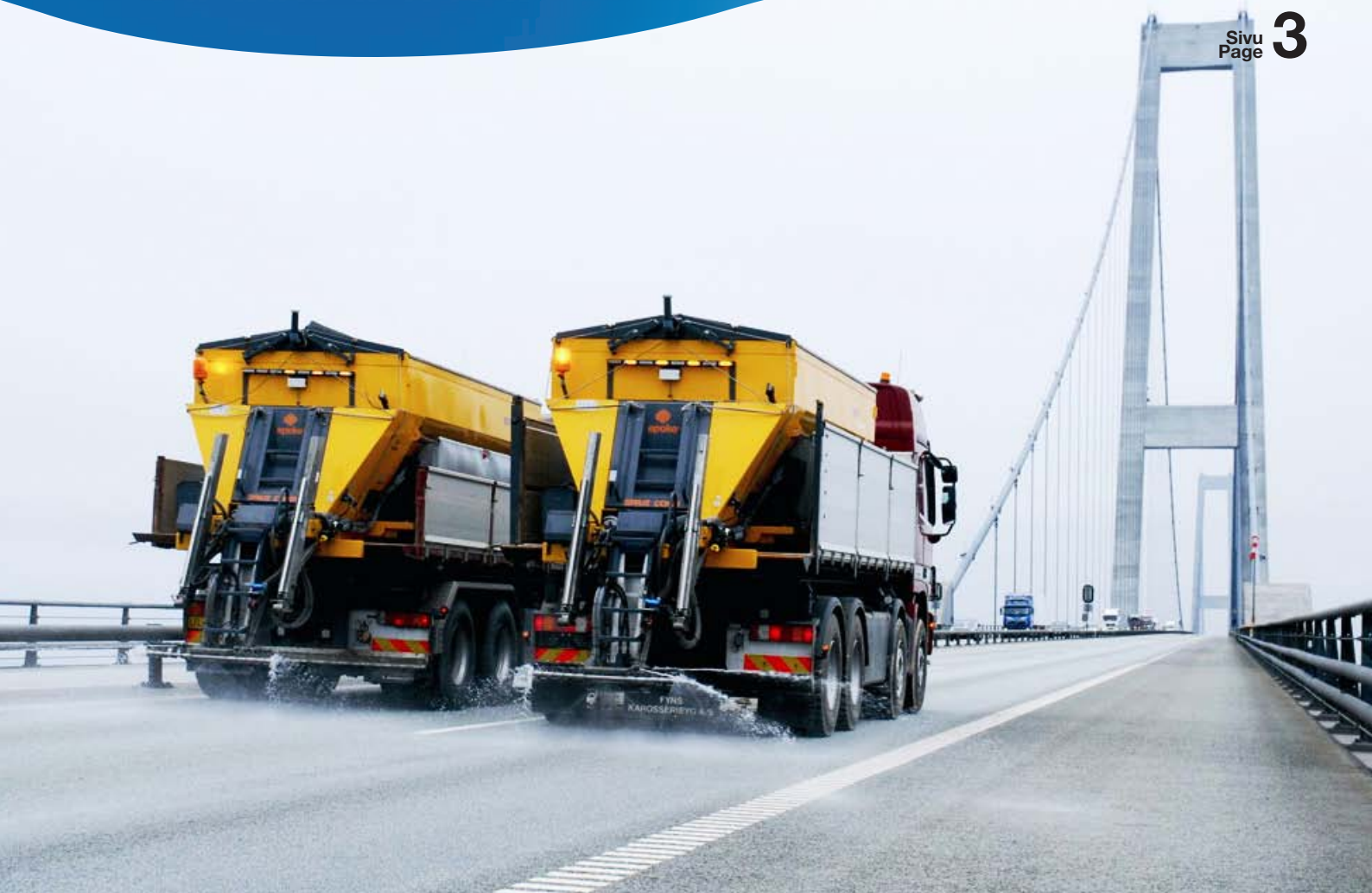
"The Great Belt Fixed Link" bridge, almost 7 km long and linking the islands of Zealand and Funen, is a major challenge when it comes to keeping the roads free of ice. The weather conditions on the bridge are the same as the sea below – a lot more extreme than on land.
