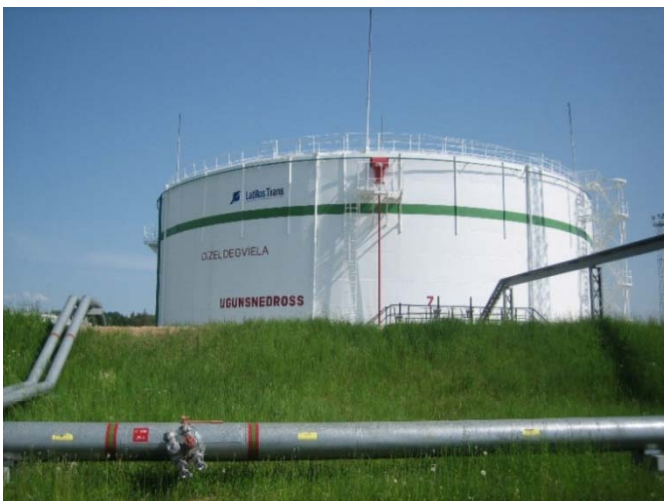
INERTA MASTIC Epoxy Coating TEKNODUR 50 Polyurethane Top Coat
